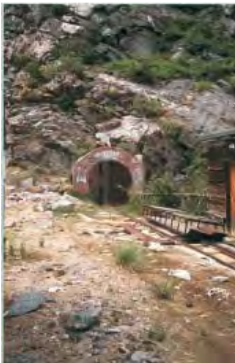
Figure 3. Burleigh Tunnel, 7/2003, photo taken by the author
